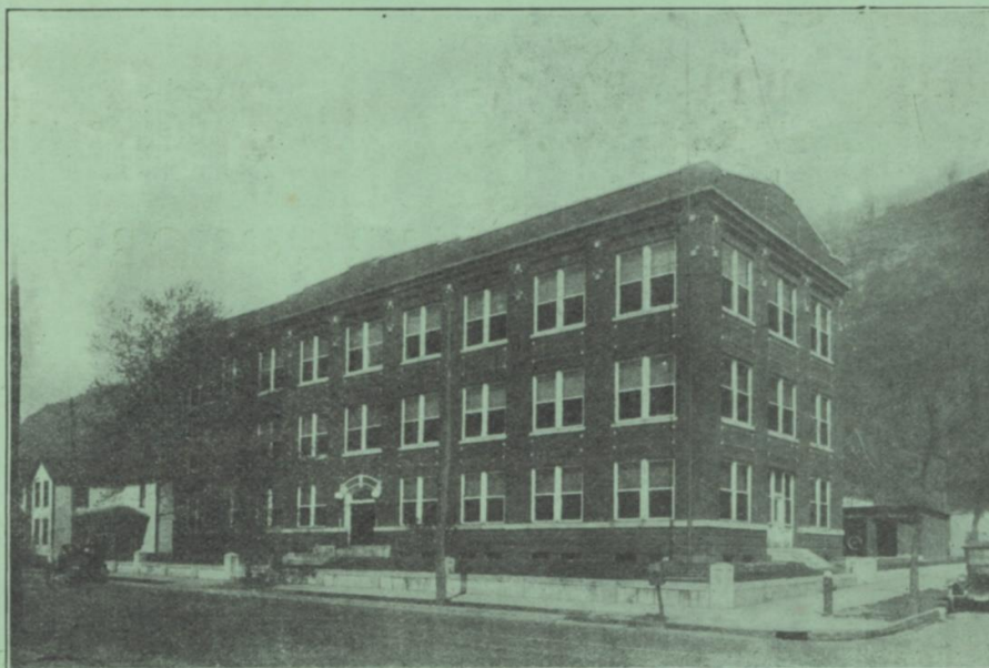
MAIN OFFICE BUILDING WHEELING STEEL CORPORATION PORTSMOUTH WORKS PORTSMOUTH, OHIO.
